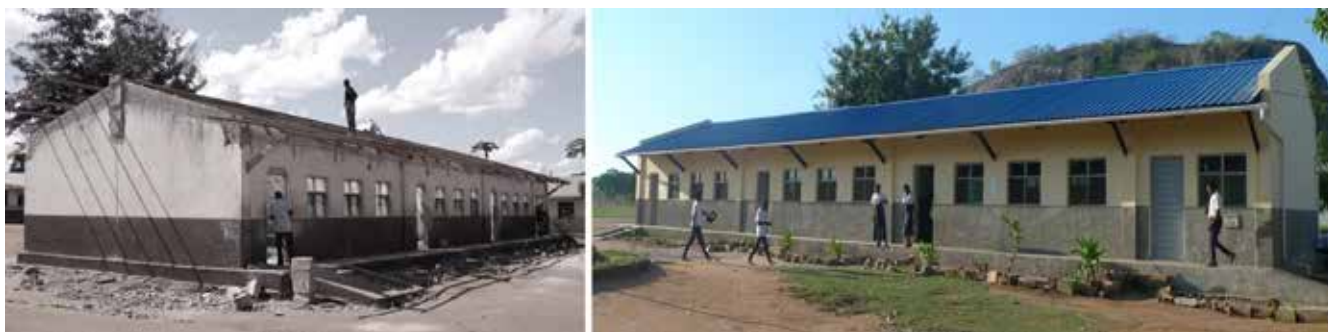
Post-disaster school reconstruction in Nampula using the methodology "Build Back Better", 2019 (photo on the right) : UN-Habitat / Juan Martinez
