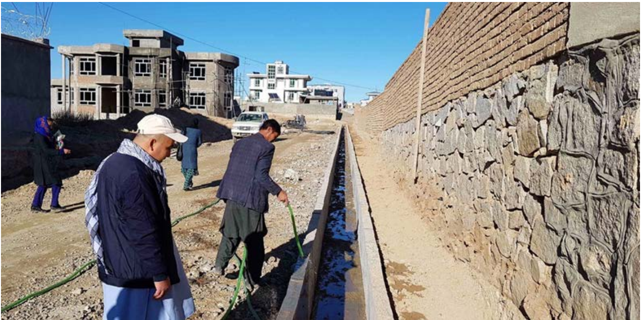
Canal Construction, Nili Province © UN-Habitat
