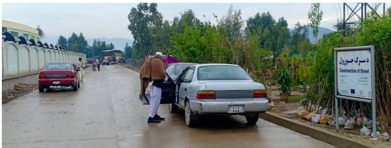
Street Construction, Jalalabad, Nangarhar Province ©Ibrahim Mohammed
