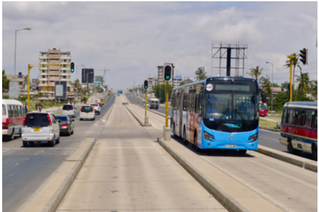
Figure 14. BRT corridor in Dar es Salaam, Tanzania.
