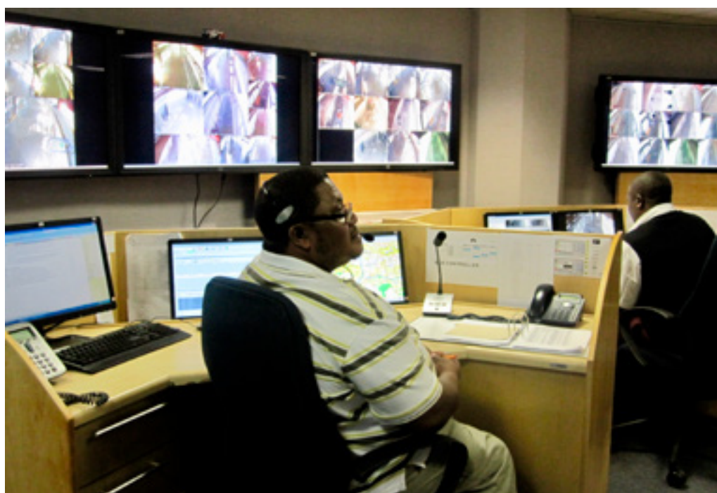
Figure 12. Control centre in Johannesburg, South Africa.
