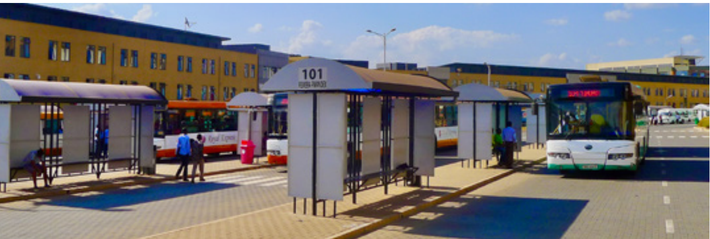
Figure 17. Bus terminal in Kigali, Rwanda.
