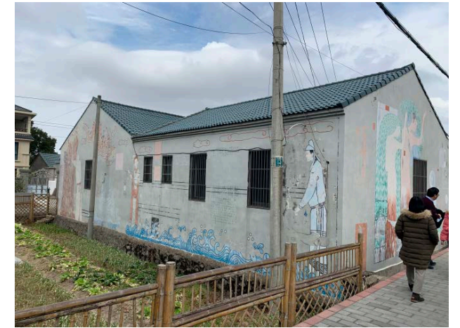
Figure 4-3-6 One-storey brick structure
