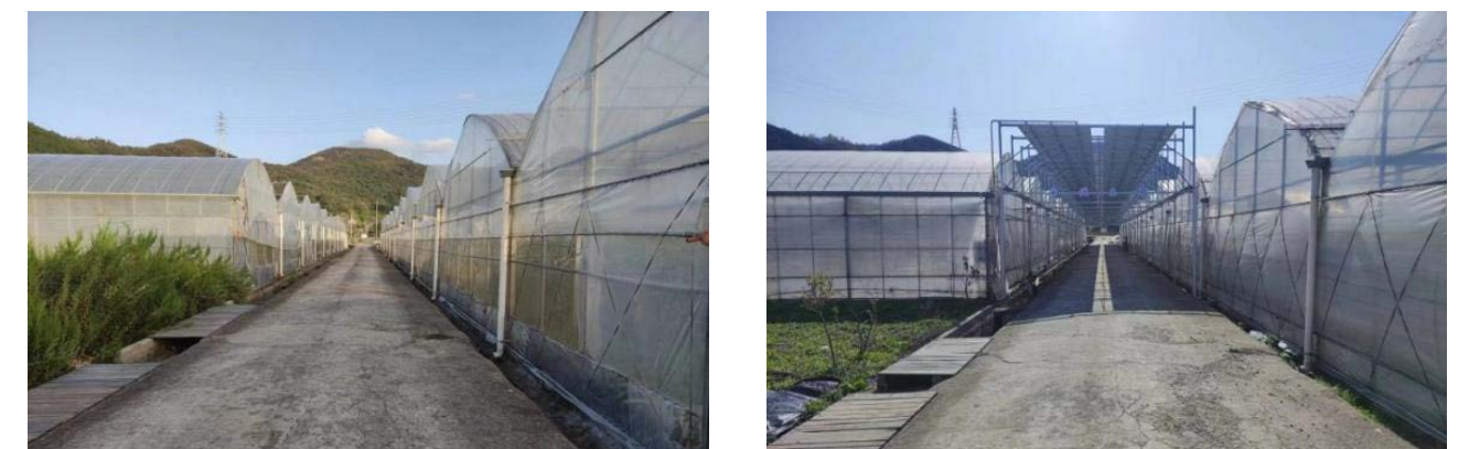
Figure 5-2-1-3 Before (left) and after (right) the installation of the photovoltaic corridor
