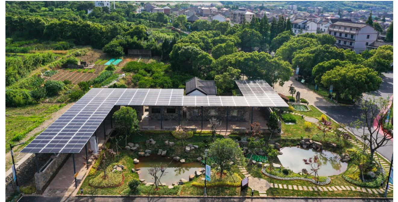
Figure 5-1-2-4 PV installed roof
