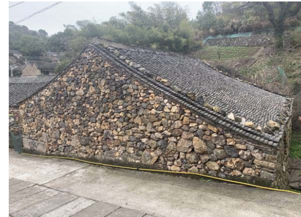
Figure 4-3-5 One-storey wood/stone structure
