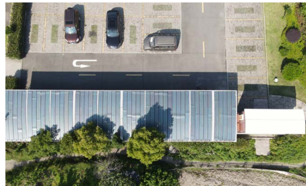
Figure 5-1-1-1 Parking lot shed with PV
