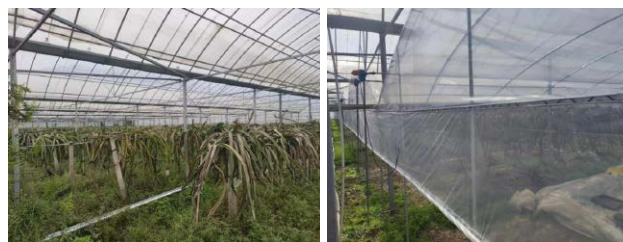
Figure 5-2-1-5 The greenhouses before (above) and after (below) the double-layer insulation renovation
