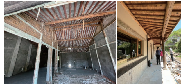
Figure 5-3-2-2 Keep the original wood-stone structure
