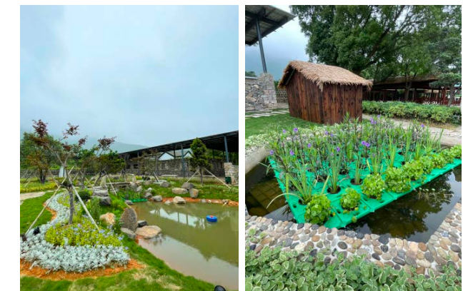
Figure 5-1-2-6 Artificial wetland for water purification
