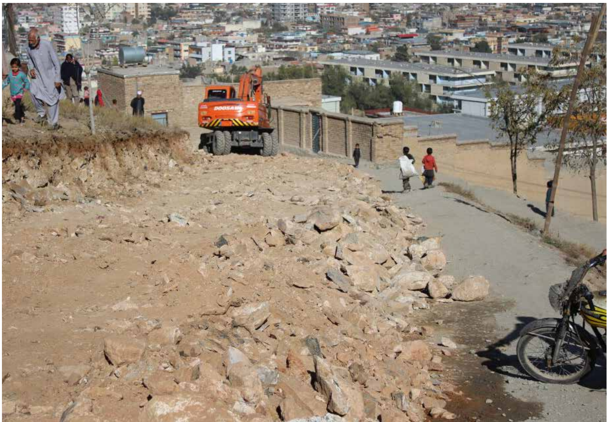
Road construction project in Kabul. Photo: Anthony Lamba
