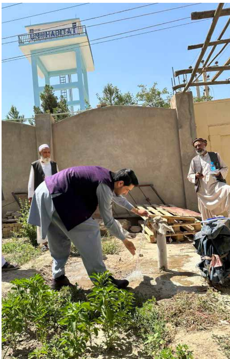
Water supply project in Mazar-i-Sharif. Photo: Anthony Lamba
