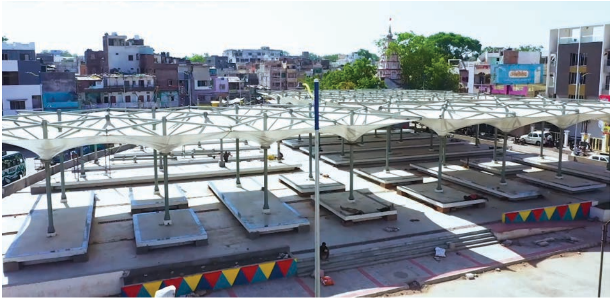
Image 6: A view of the transformed Jinsi Market in Indore. The redeveloped market today provides employment to over 1,000 persons each day, according to ISCDCL. Source: Indore Smart City
