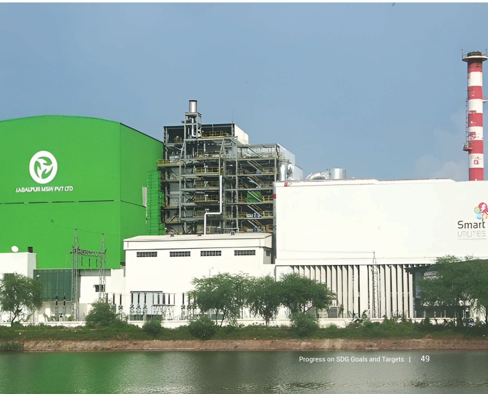
Image 20: A first-of-its-kind Waste-to-Energy plant developed in PPP mode in Jabalpur employs mass burning technology, incinerating 600 tonnes of old, new, and unsorted waste while adhering to industrial standards and regulatory requirements. The plant generates around 11.5 MW of electricity daily, which is sold to the Madhya Pradesh Electricity Board (MPEB). Source: Jabalpur Smart City.
