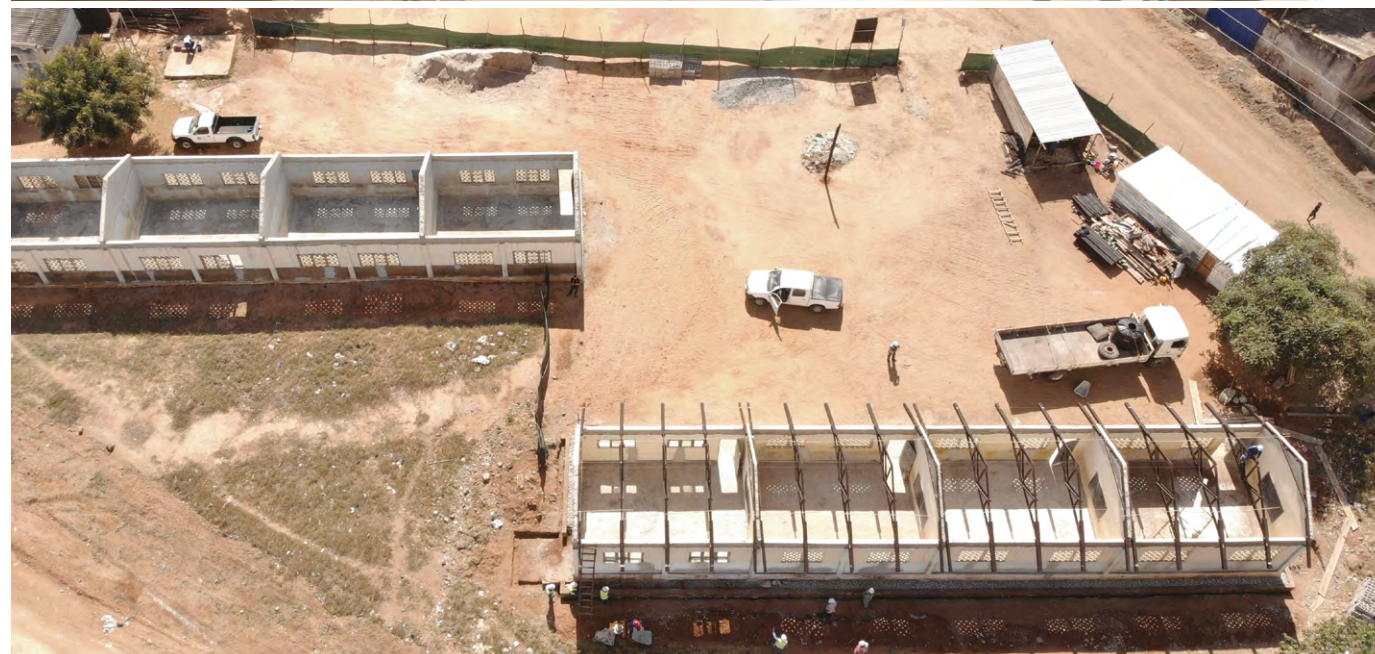
Monapo School, Nampula Province - Reconstruction Process | Source: UN-Habitat
