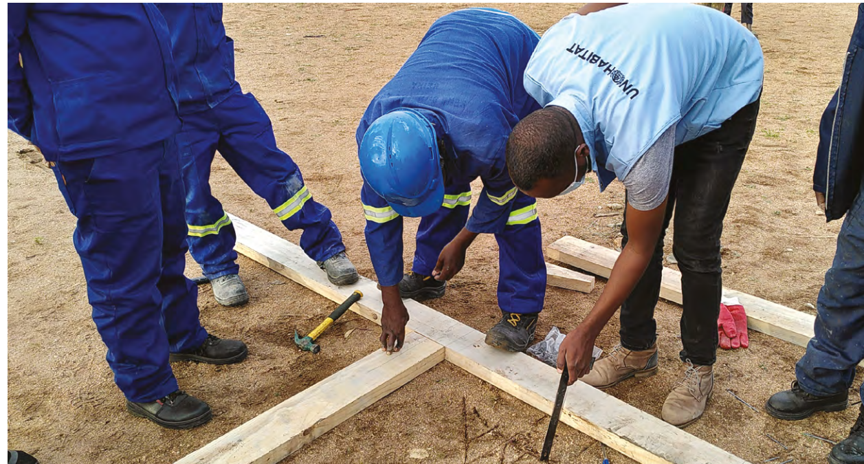
On-the-job training on resilient school construction. Sofala 2022
