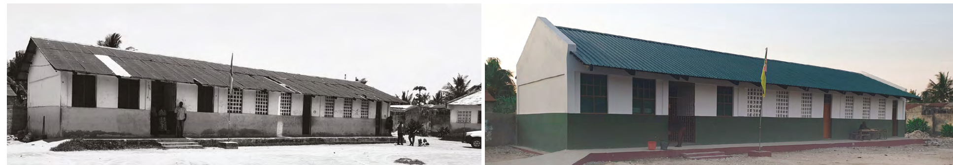
Torrone Velho School - before and after reconstruction process | Source: UN-Habitat
