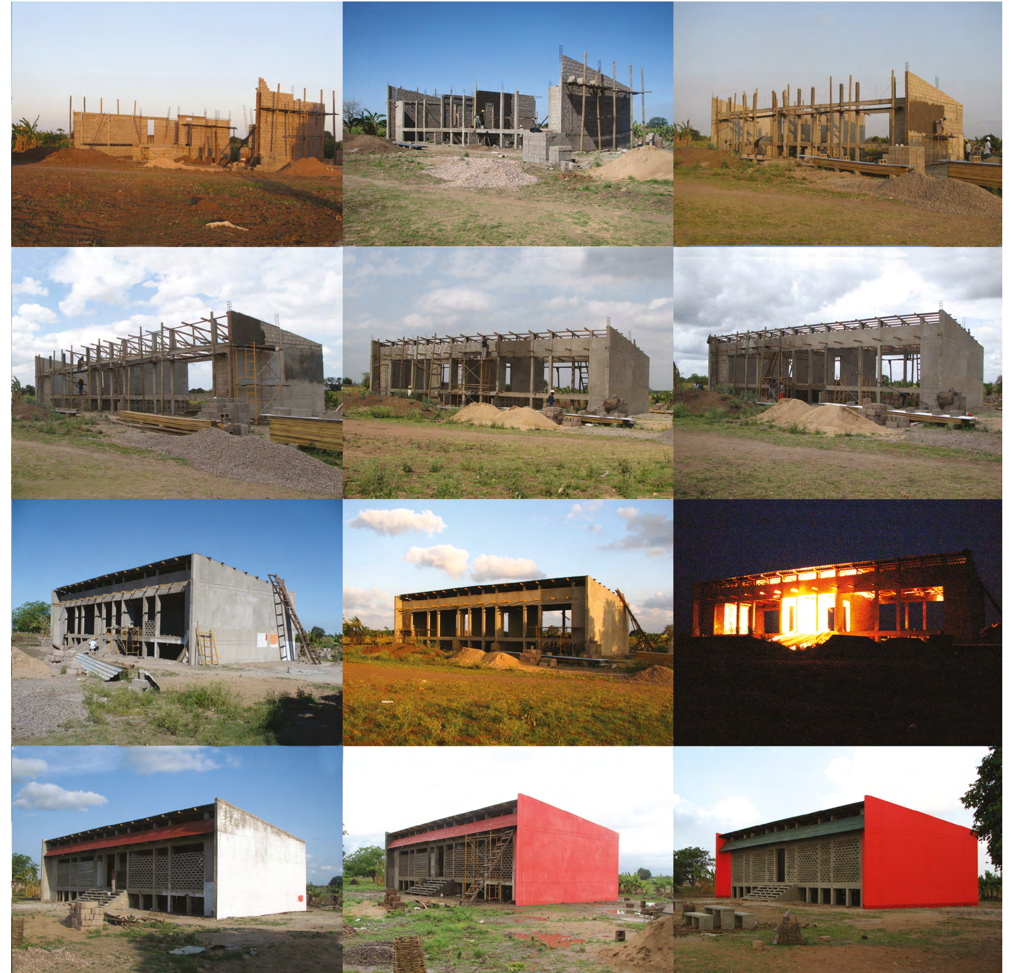
Maniquenique School construction process | Source: UN-Habitat
