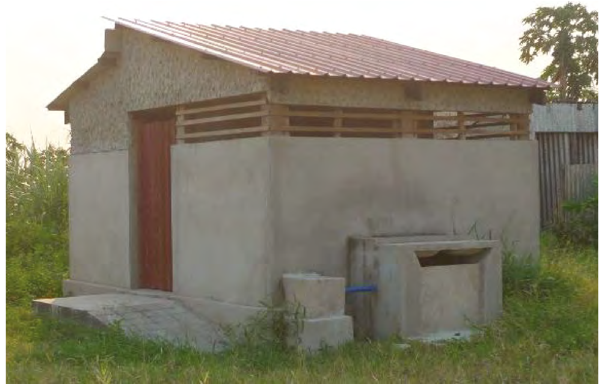
Mazoao School - Reconstruction Process | Source: UN-Habitat
