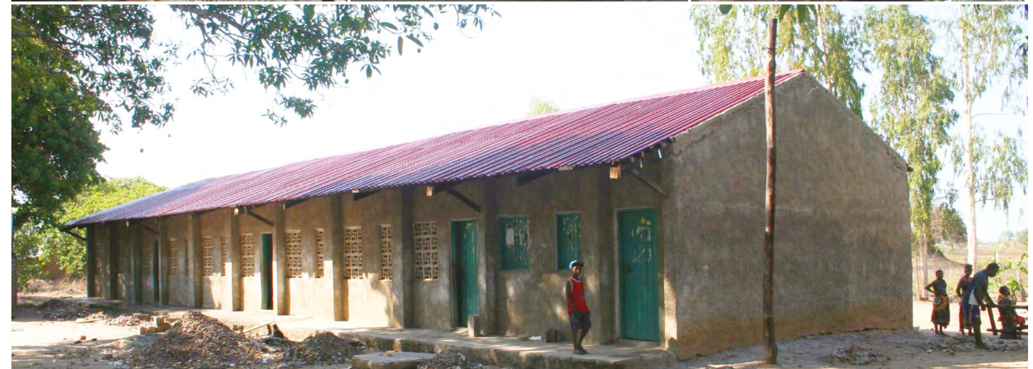
Primary School " 4 de Outubro" - Rehabilitation Process | Source: UN-Habitat
