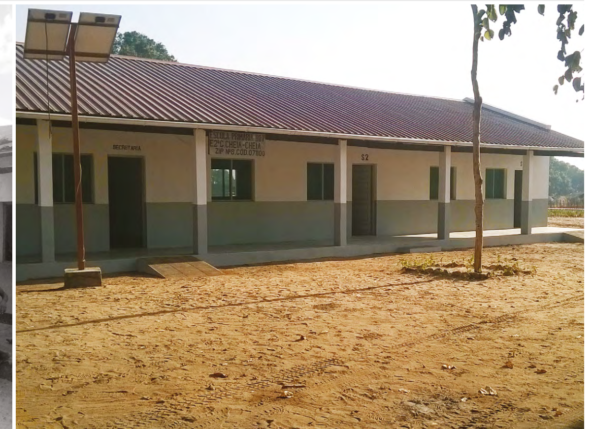
Cheia-Cheia School, Niassa Province - Before and After reconstruction | Source: UN-Habitat
