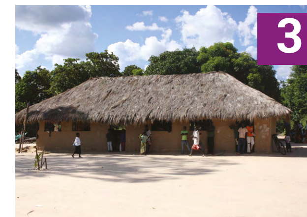
Typical Local Materials School | Source: UN-Habitat
