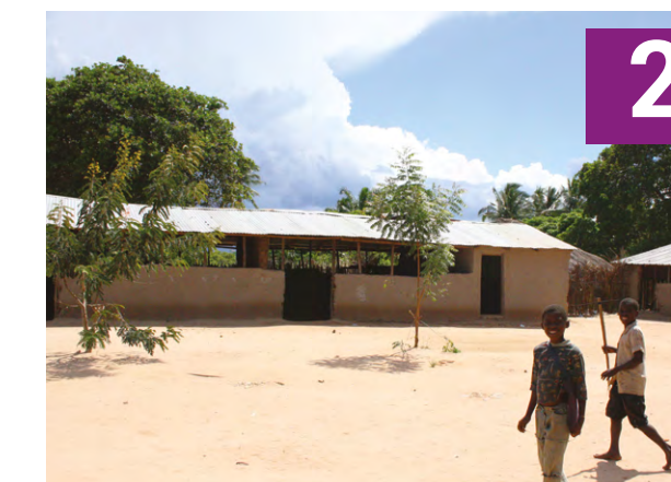
Typical Mixed Materials School | Source: UN-Habitat
