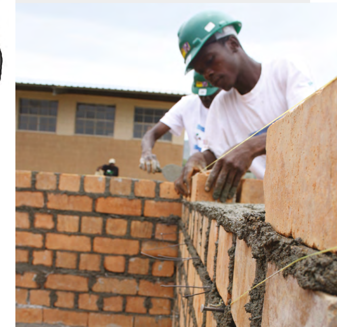
Training on Earthquake Resistant Construction using bamboo slats | Source: UN-Habitat
