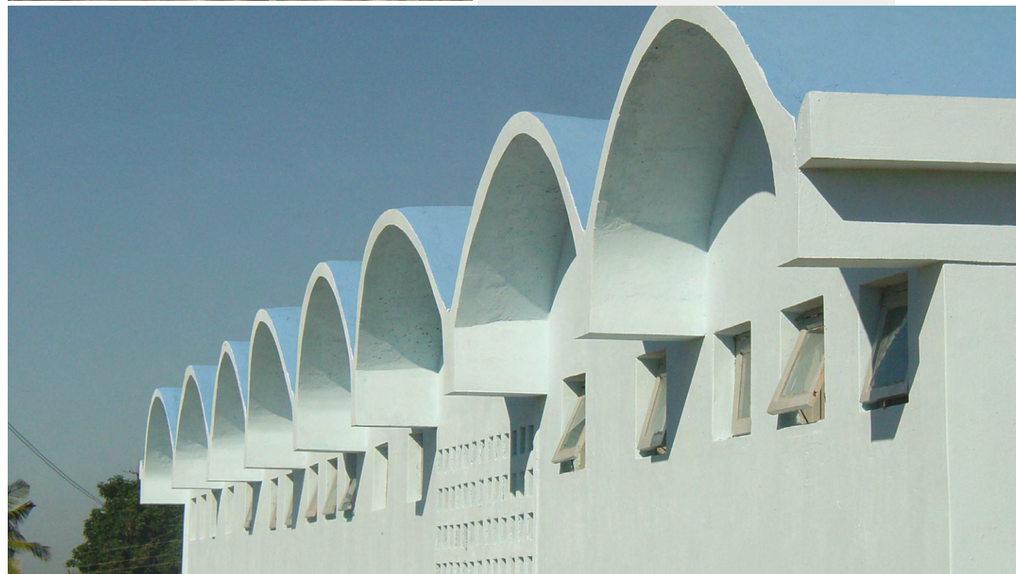
School innovative roofing system | Source: UN-Habitat
