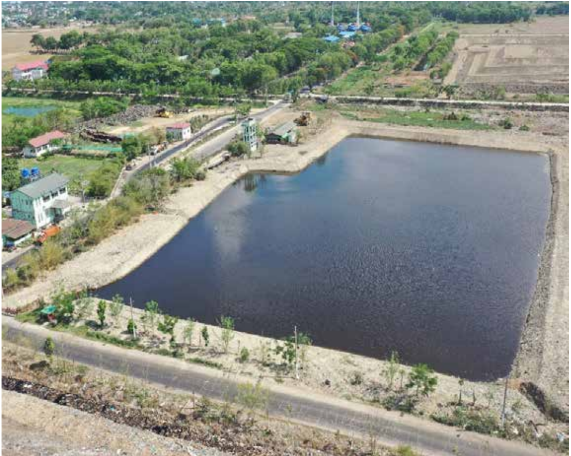
Leachate collection pond in Htein Bin FDS © UN-Habitat
