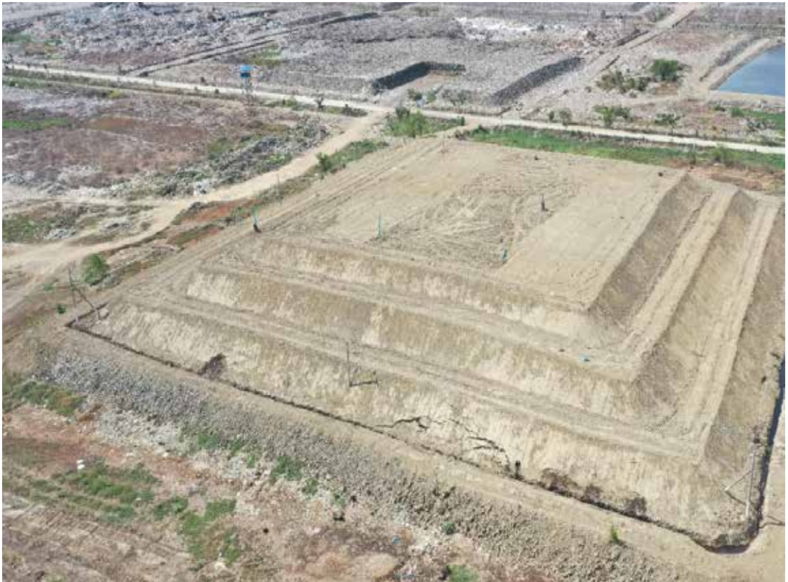
Completed landfill cell of Fukuoka method at Htein Bin FDS © UN-Habitat
