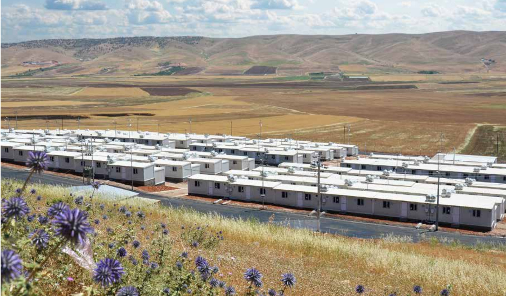
IDP Shelter Site.in Iraq @UN-Habitat
