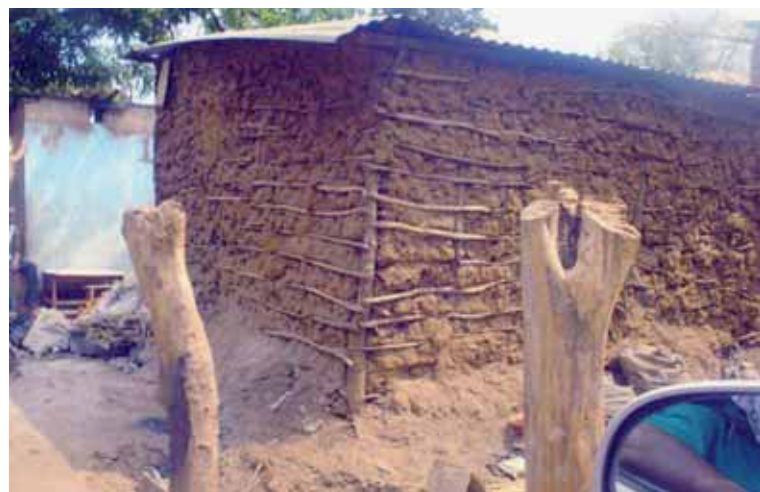
Figure 69. Pole and dagga walling, Livingstone. Photo © UN-Habitat/Daniel Phiri
