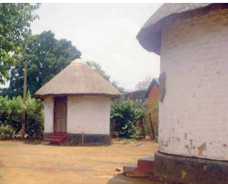
Figure 29. Old Kabwata dwellings restored to original condition. Photo © UN-Habitat
