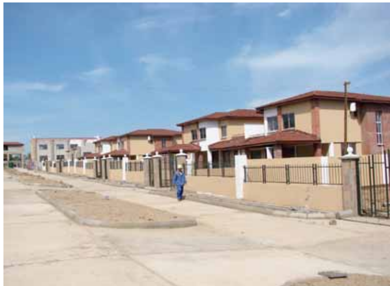
Figure 15. NHA and NAPSA housing at Leopard's Hill, Lusaka. Photo © UN-Habitat
