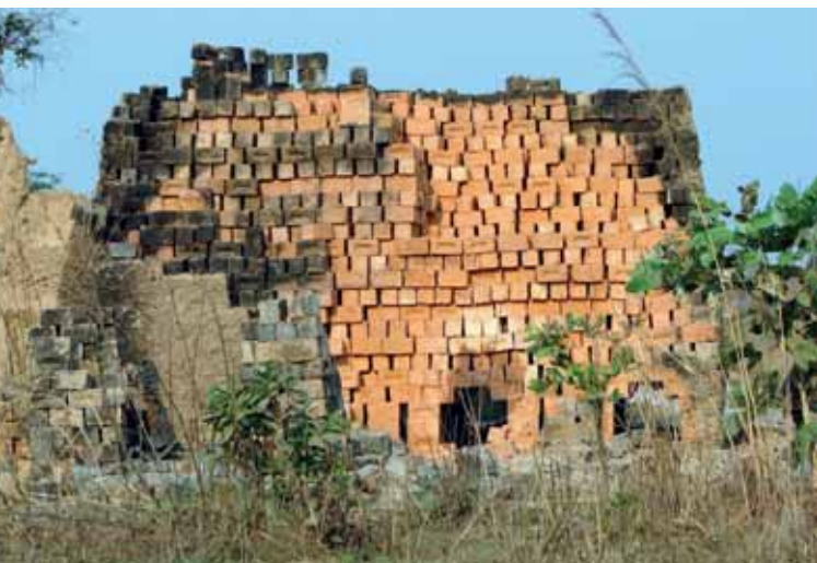
Figure 78. Brick making from anthill soil, Kitwe. Photo © UN-Habitat
