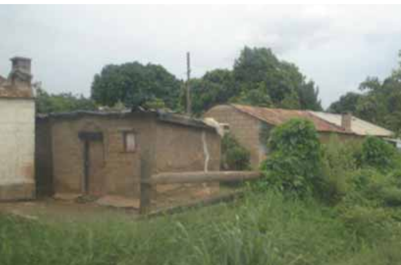
Figure 87. Small rental dwelling added on a plot in Buchi, Kitwe. Photo © UN-Habitat/Daniel Phiri
