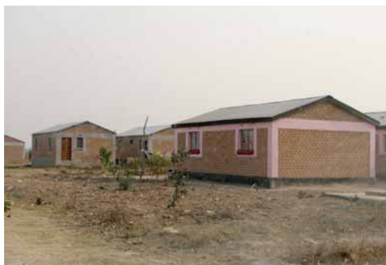
Figure 81. Dwellings built with Hydraform blocks, Kawama, Kitwe. Photo © UN-Habitat
