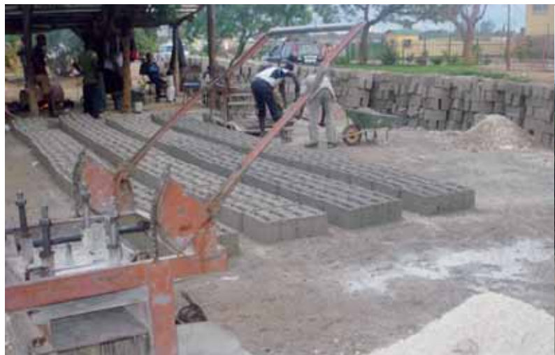
Figure 77. Informal manufacture of cement blocks, Kalingalinga, Lusaka. Photo © UN-Habitat
