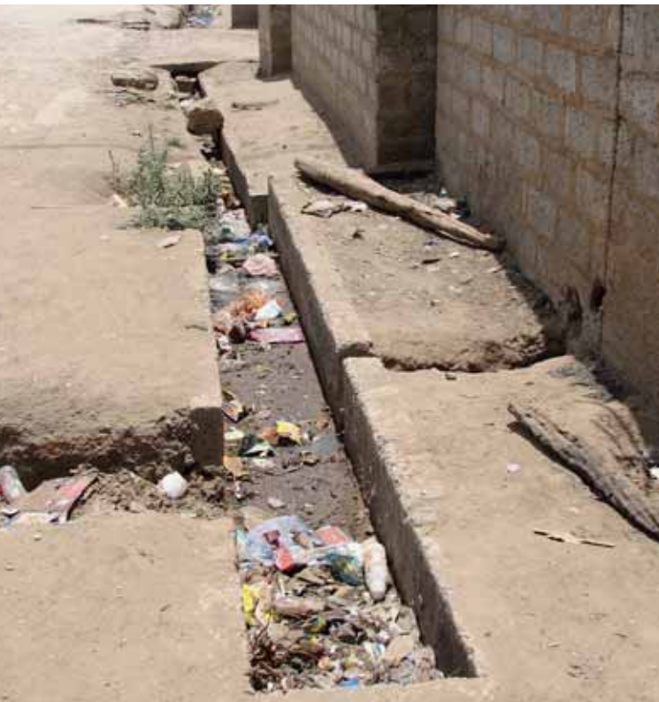
Figure 63. Self-help drains in Garden, Lusaka. Photo © UN-Habitat
