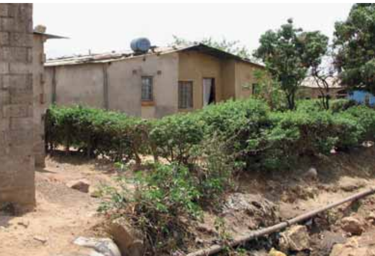
Figure 70. Good quality informal sector housing, Chaisa, Lusaka. Photo © UN-Habitat
