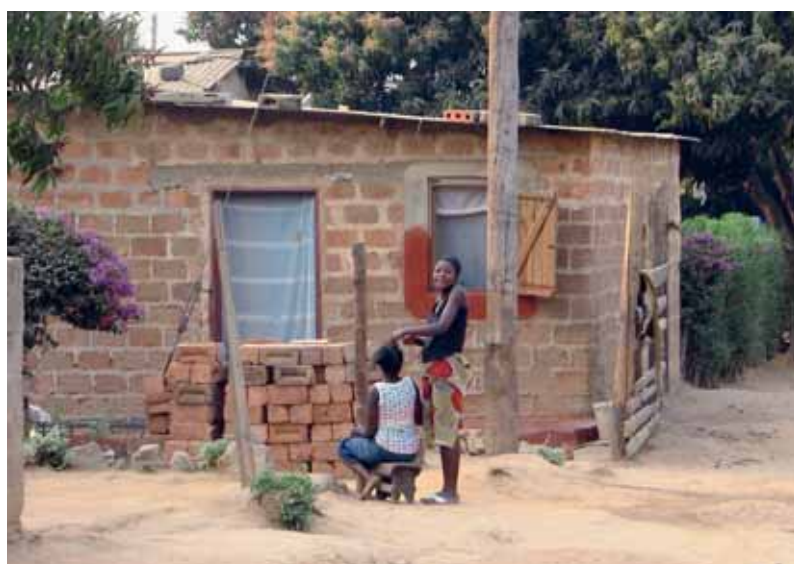
Figure 37. Soil-cement block house in Kamatipa informal settlement, Kitwe. Photo © UN-Habitat
