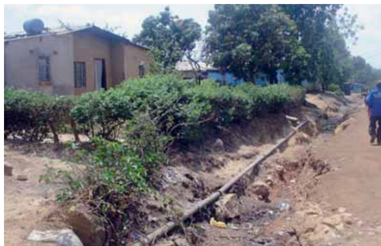
Figure 52. A water main fitted in Chaisa, Lusaka. Photo © UN-Habitat/Daniel Phiri
