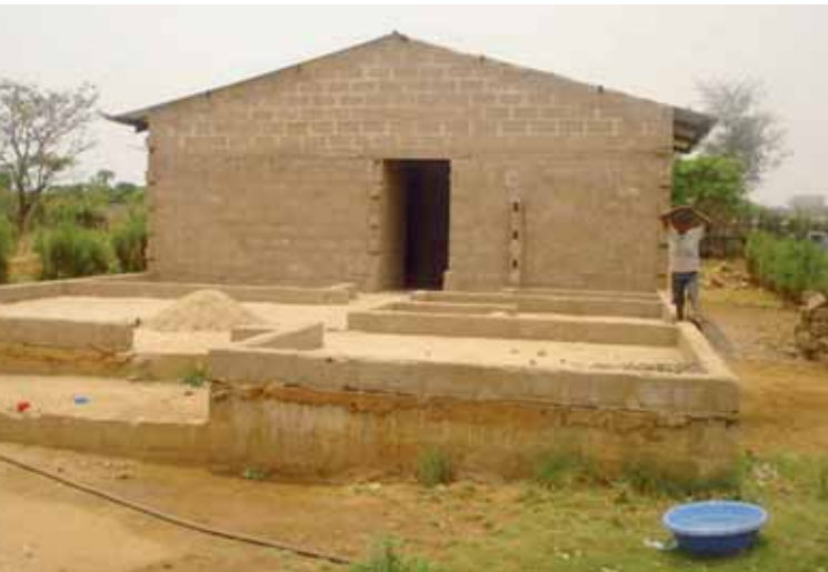
Figure 65. The incremental building process, Dambwa, Livingstone. Photo © UN-Habitat/Daniel Phiri
