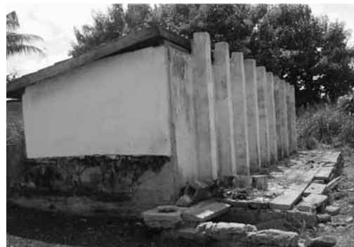
Picture 7: Toilet facility in the Control Community
