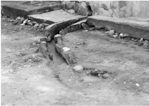
Picture 6: Waste water from a bathhouse in the Control Community
