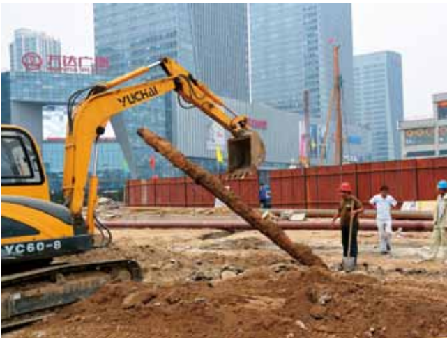
Water Pipeline Renovation in Langfang City (Photo by Li Zonglai)
