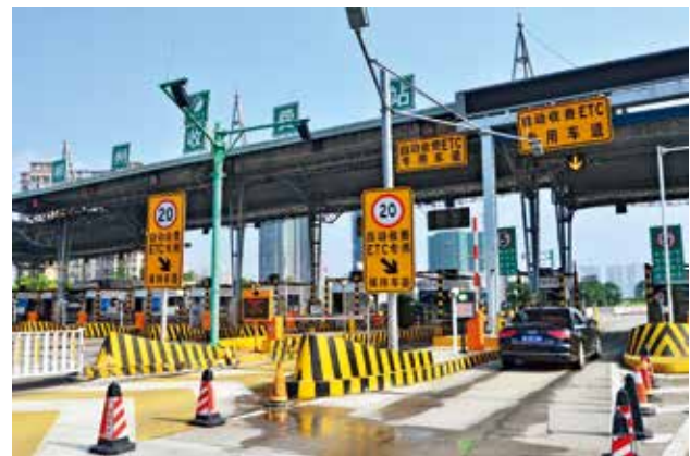
Figure 1-14 ETC lane in Chenzhou Toll Gate along Beijing-Hong Kong-Macau Expressway (Photo taken by He Maofeng)
