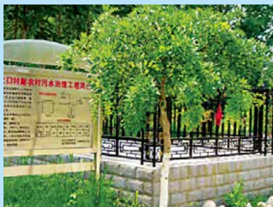
Sewage treatment system built for each village
