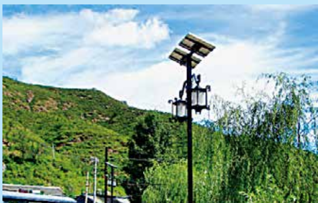
Energy-saving lights installed on main roads of all villages
