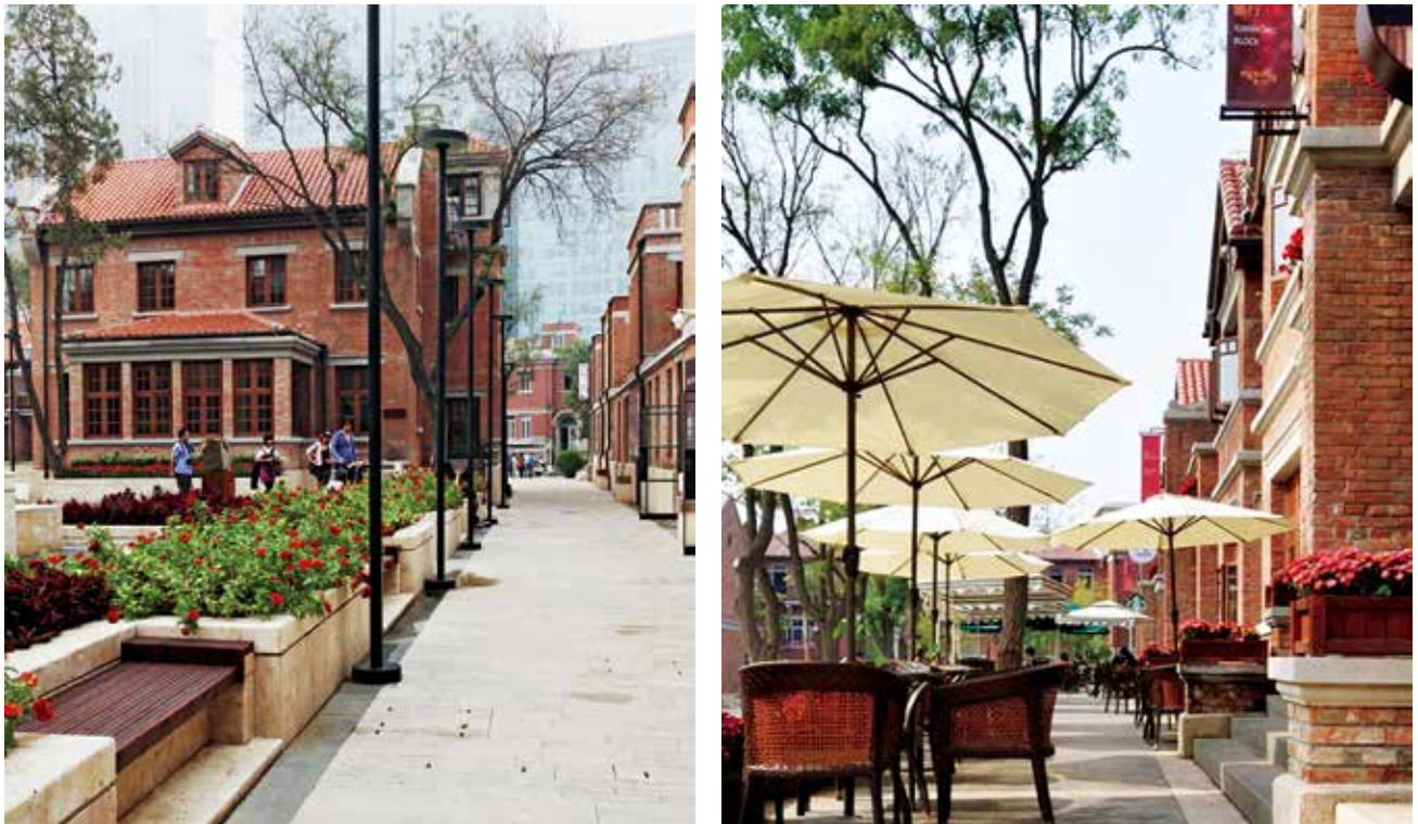
Figure 6-13 Pictures for current state of No. 24 housing block after implementing the protection and renewal planning (Source: Research on Protection and Renewal Planning of Historical and Cultural Blocks, Five-Avenue, Tianjin, China )
