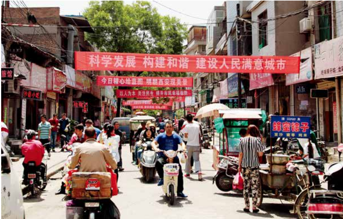
Figure 2-35 Xi'an: Last moment visit to the largest shanty area to be demolished (Photo by Zhang Yuan)
