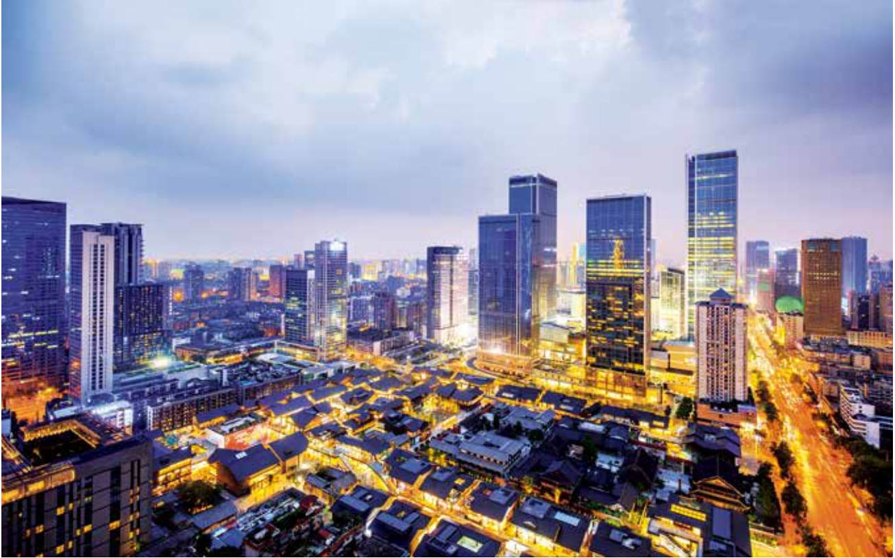
Figure 6-20 Bird's eye view of night scene of Sino-Ocean Taikoo Li Chengdu (Photo by Wei Fenggao) (Source: www.huitu.com)
